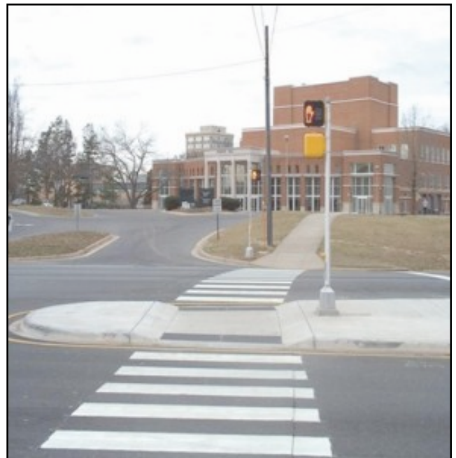
Median Refuge Island
